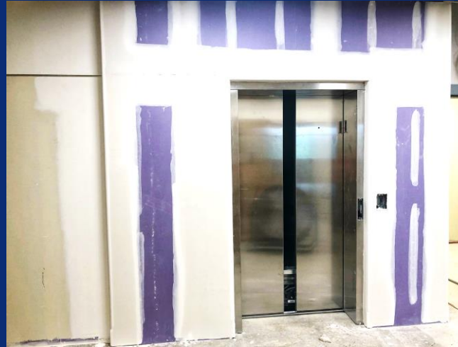
Elevator Door Installation 3 rd Level
