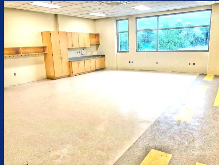
Millwork and VCT Installed 2 nd Level West
