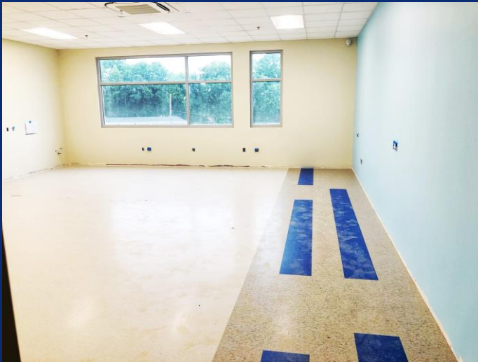
VCT and Accent Wall Paint Installed 3 rd level West
