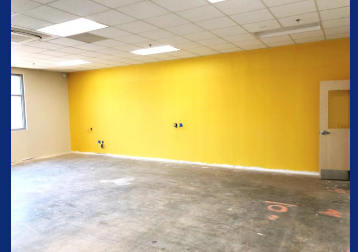
ACT Installed at 2 nd Level East Classrooms
