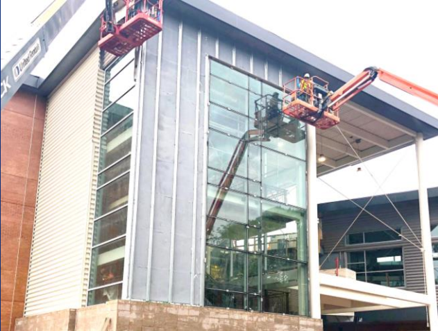
South Stair Tower Metal Panel and Curtain Wall
